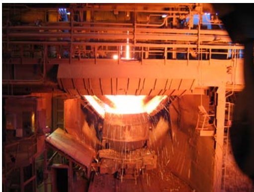
Fig. 3. Photograph of the discharge installation located in the steelworks
